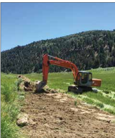
Working on ranch improvements.
