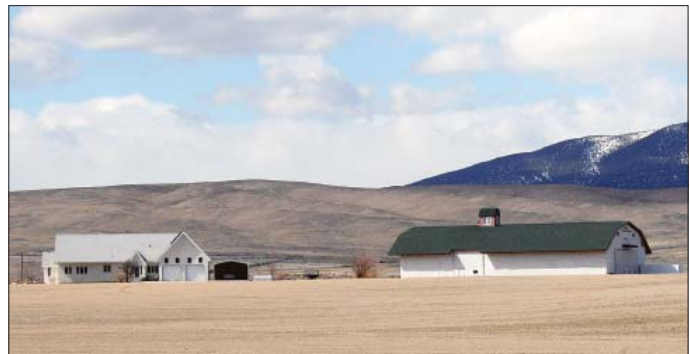
The Tuft's home and the barn made of stuccoed straw bales.
